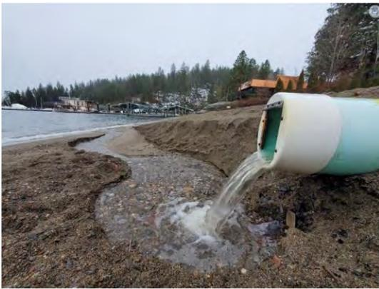
Figure 7. Uncontrolled stormwater outflow causing beach erosion.
